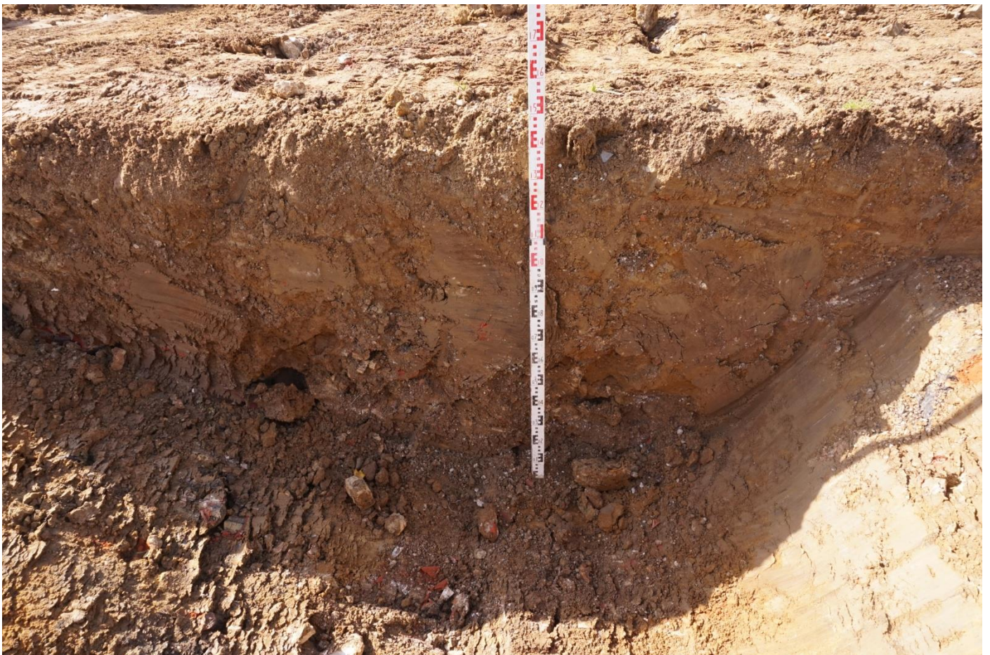
Plate 6: Looking west at 1.5m deep test pit in trench 3 through modern hardcore/clay deposit. No natural exposed within the trench
